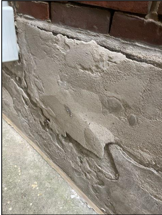
Parging damaged or missing
