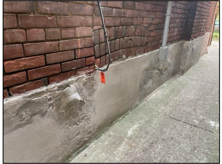
Parging damaged or missing
